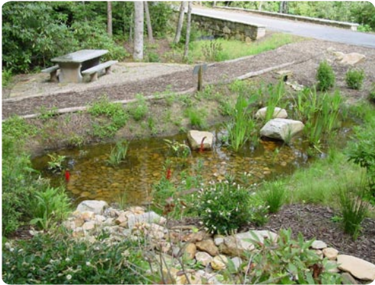
Constructed wetlands used as a stormwater management control measure
