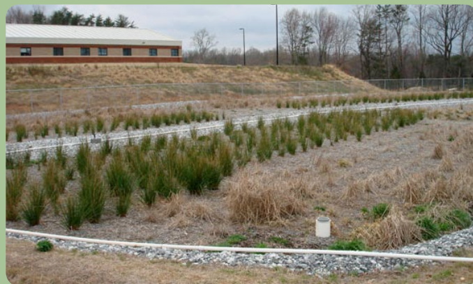
Constructed wetland that is part of the Living Machine® wastewater treatment system at North Guilford Middle School in Guilford County, NC. The system saves 5 million gallons of water per year by reusing treated water for irrigation. (Worrell Technologies)
