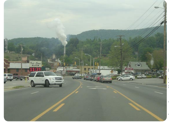
Lack of access control in Sylva, NC along NC 107 results in unpredictable turning movements and dangerous conditions for motorists, pedestrians, and cyclists.
