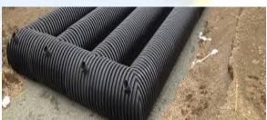
**Purpose:** underground stormwater detention systems manage and control the volume and discharge timing of stormwater runoff.
