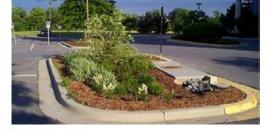
and bacteria from the stormwater runoff). It can also be used to reduce peak runoff rates and increase stormwater infiltration. In a nutshell, a bio cell is designed to hold and filter water.
