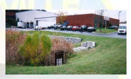
**FILTER STRIPS** are gently sloping, vegetated areas adjacent to impervious surfaces. Sometimes referred to as vegetated filter strips, grassed filter strips, grassed filters, or buffer strips, they help remove sediments, other pollutants and increase infiltration. Originally developed as an agricultural treatment practice, filter strips have now become a common urban stormwater management practice.
