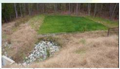
**Purpose:** They are intended to reduce impacts of sheet flow and velocity of stormwater and help improve its water quality.
