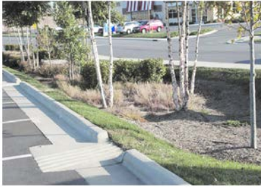
Example of discontinuous curbing around parking lot bio-retention area
