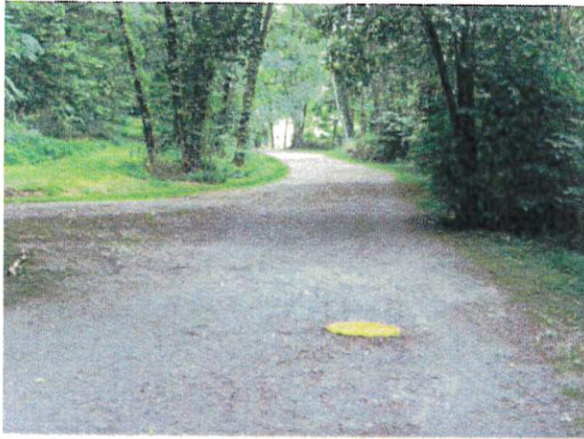
Above: Utility access points, as shown above on the Virginia Creeper Trail, can be highlighted with paint when creating a flush transition to a trail is difficult due to existing design features.
