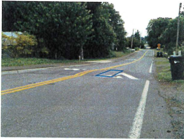
These speed humps are designed to allow both emergency vehicles and bicyclists to travel through them without impeding their speed (gap highlighted in blue).
