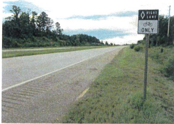
Below: Rumble strips along US 27 in south Georgia allow space for bicyclists to operate along the shoulder. Georgia also recommends gaps in the rumble strips at regular intervals.
