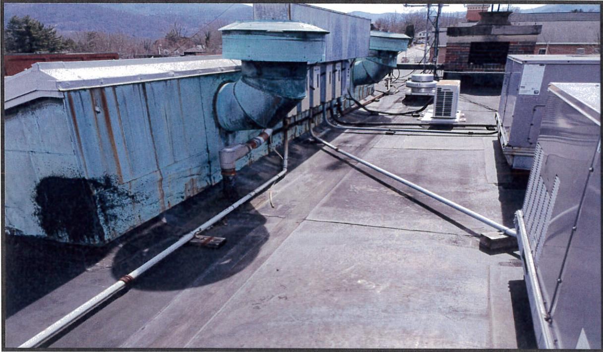
**Water has got between the walls and the material causing the parapet wall to pull apart making a water pocket.**
