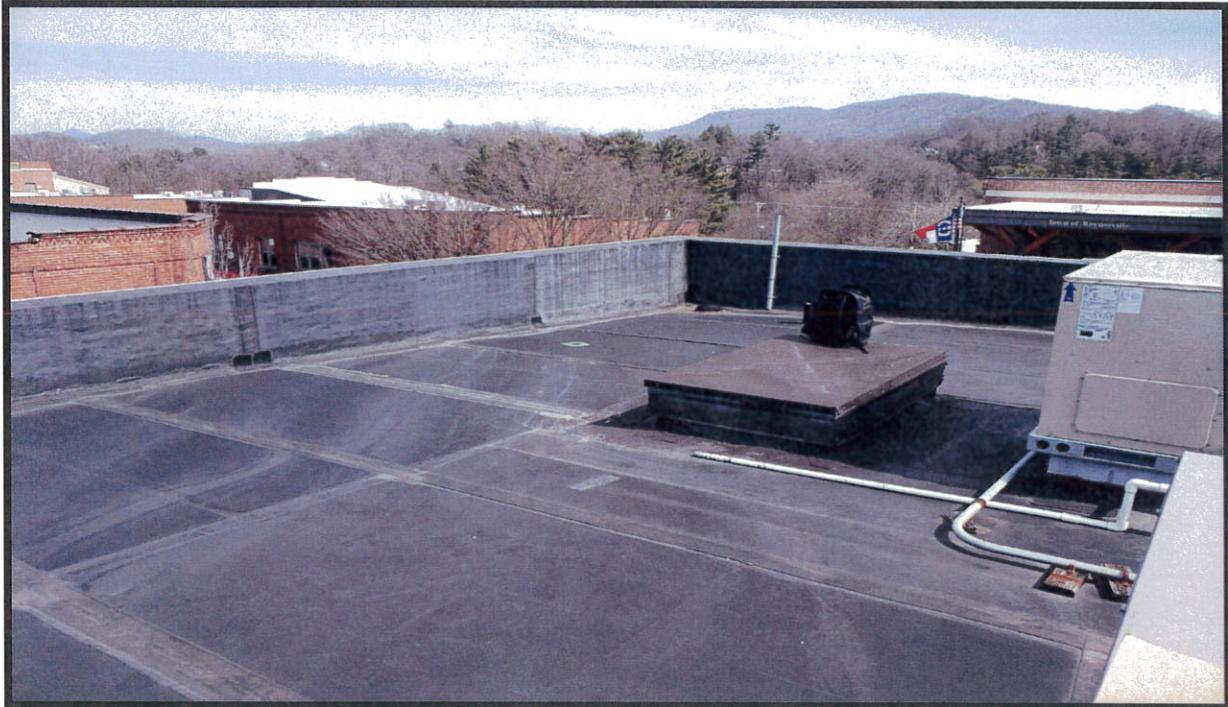
**With the age of the roof it is starting to pull apart from the seams allowing water to travel throughout the roof.**
