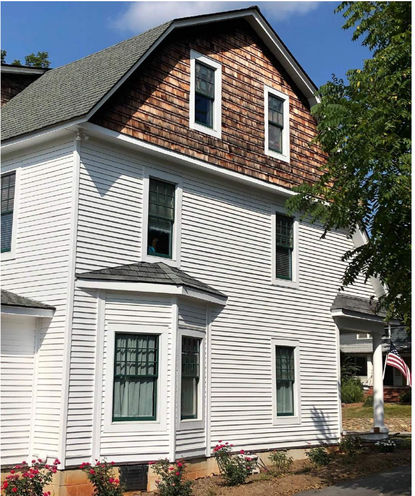
View from South Side
