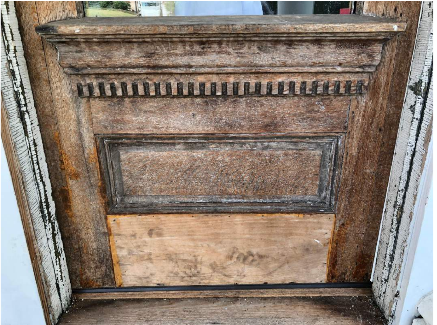
Front Entrance Door – Lower Detail
