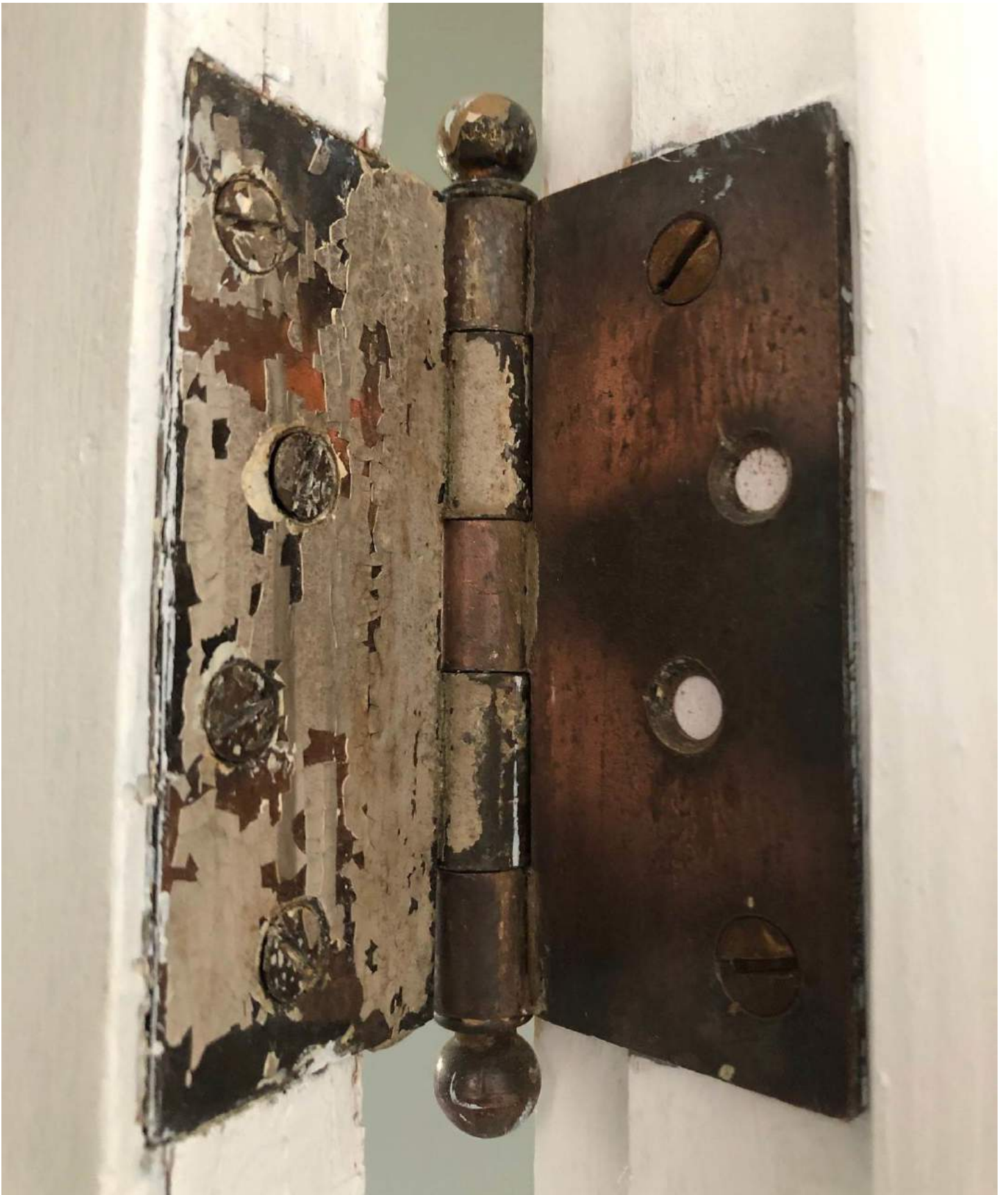
Original Door Hinge – Found on Most Doors Throughout
