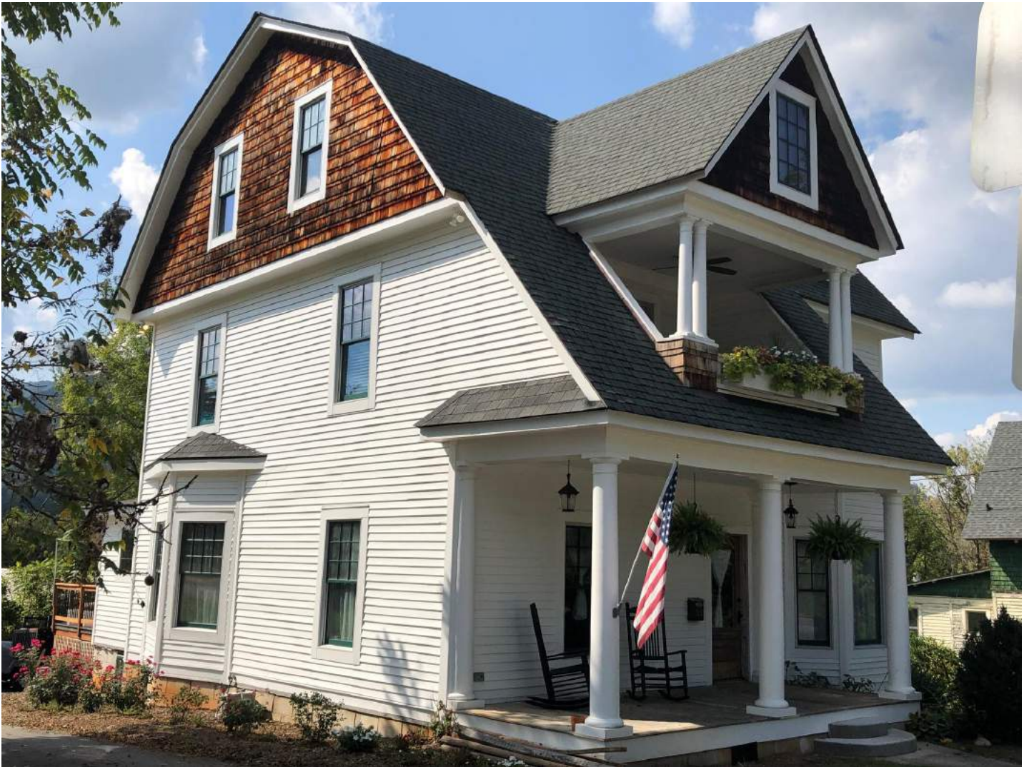
View from Southeast Corner
