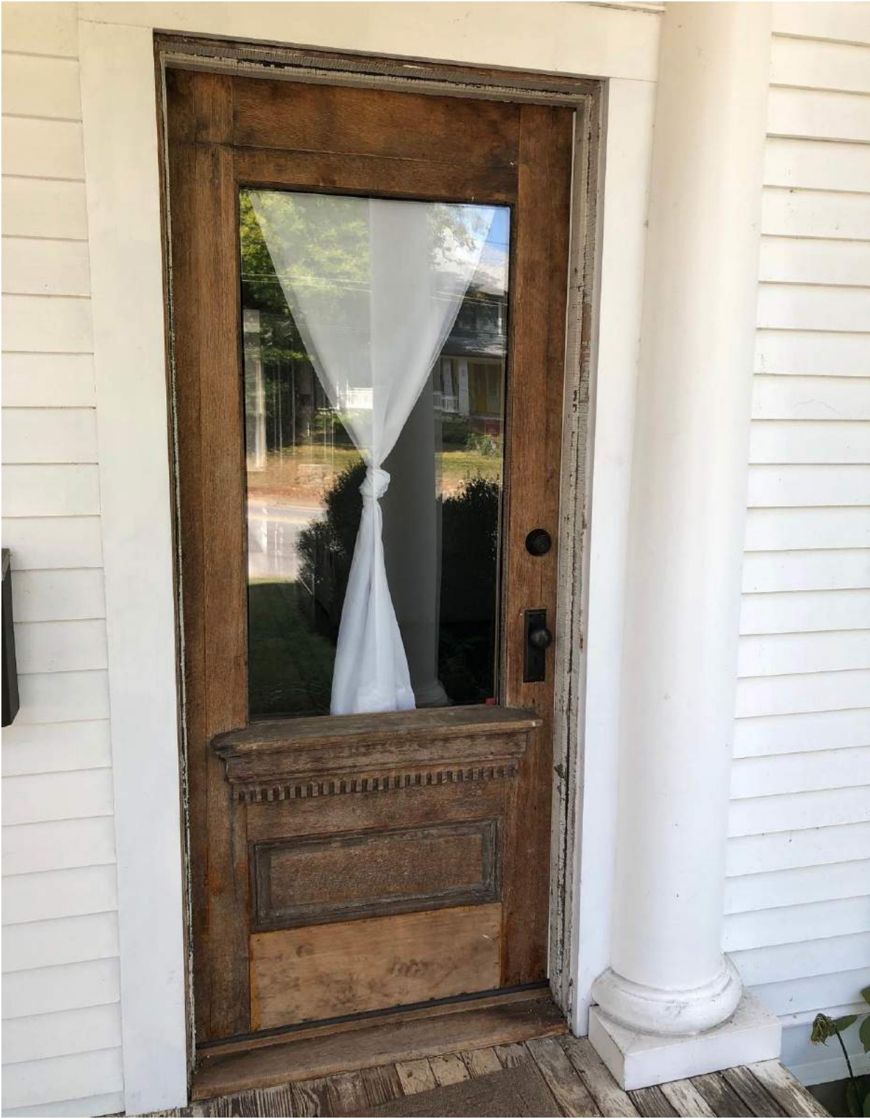
Front Entrance Door
