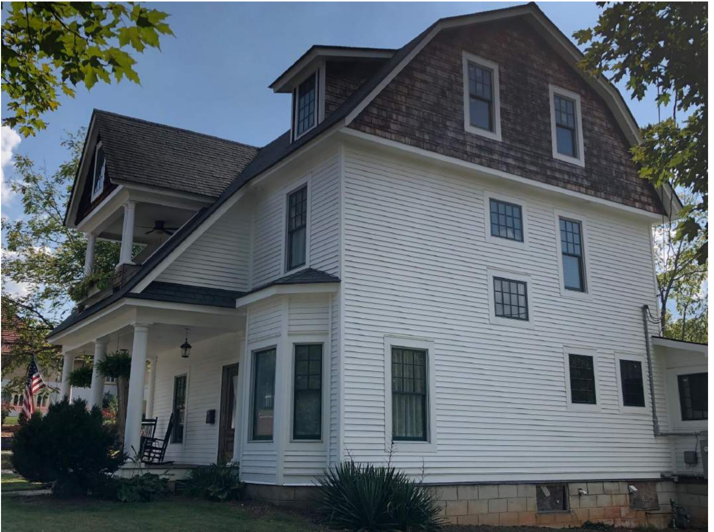
View from Northeast Corner
