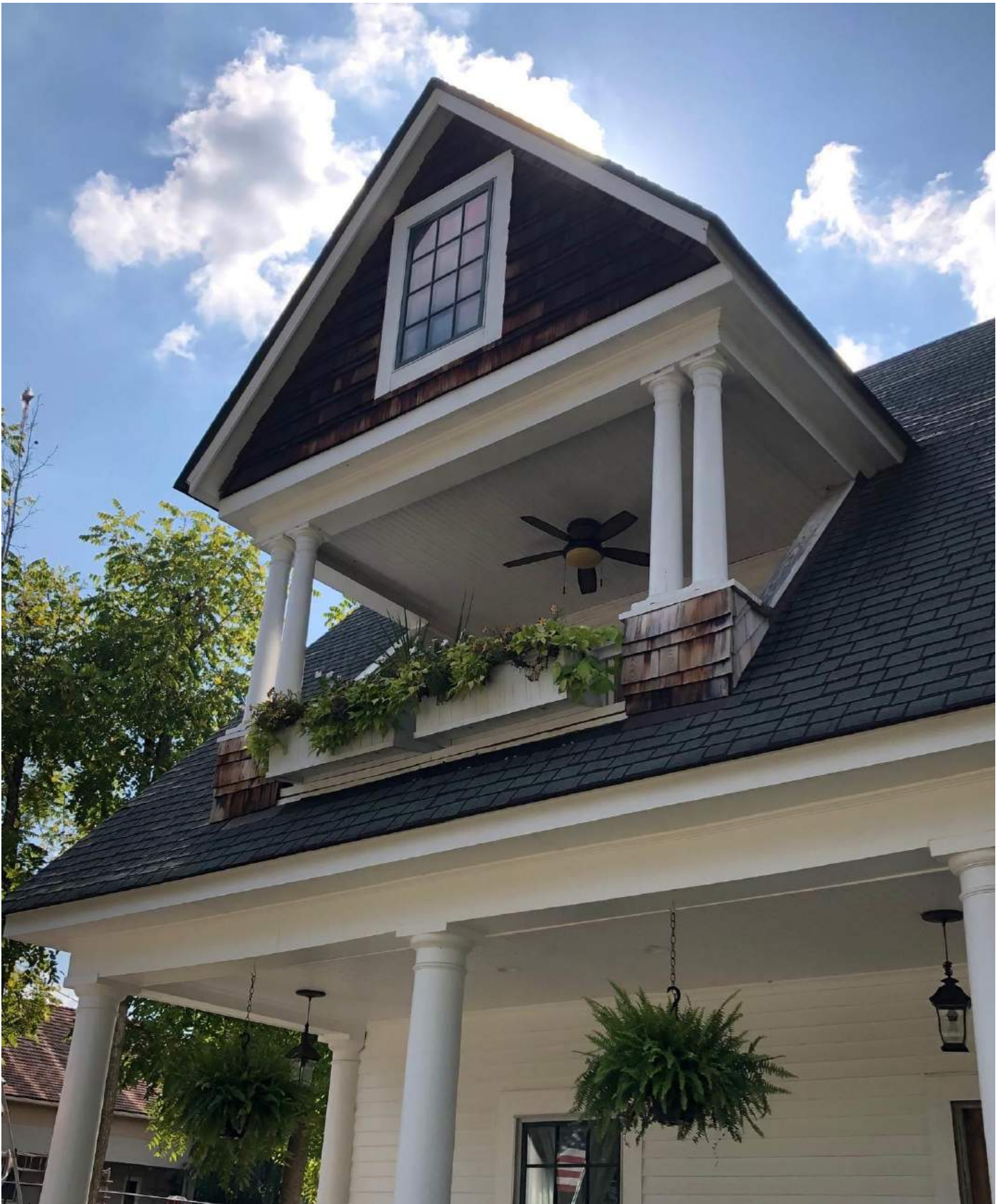
Second-Story Porch from East Side
