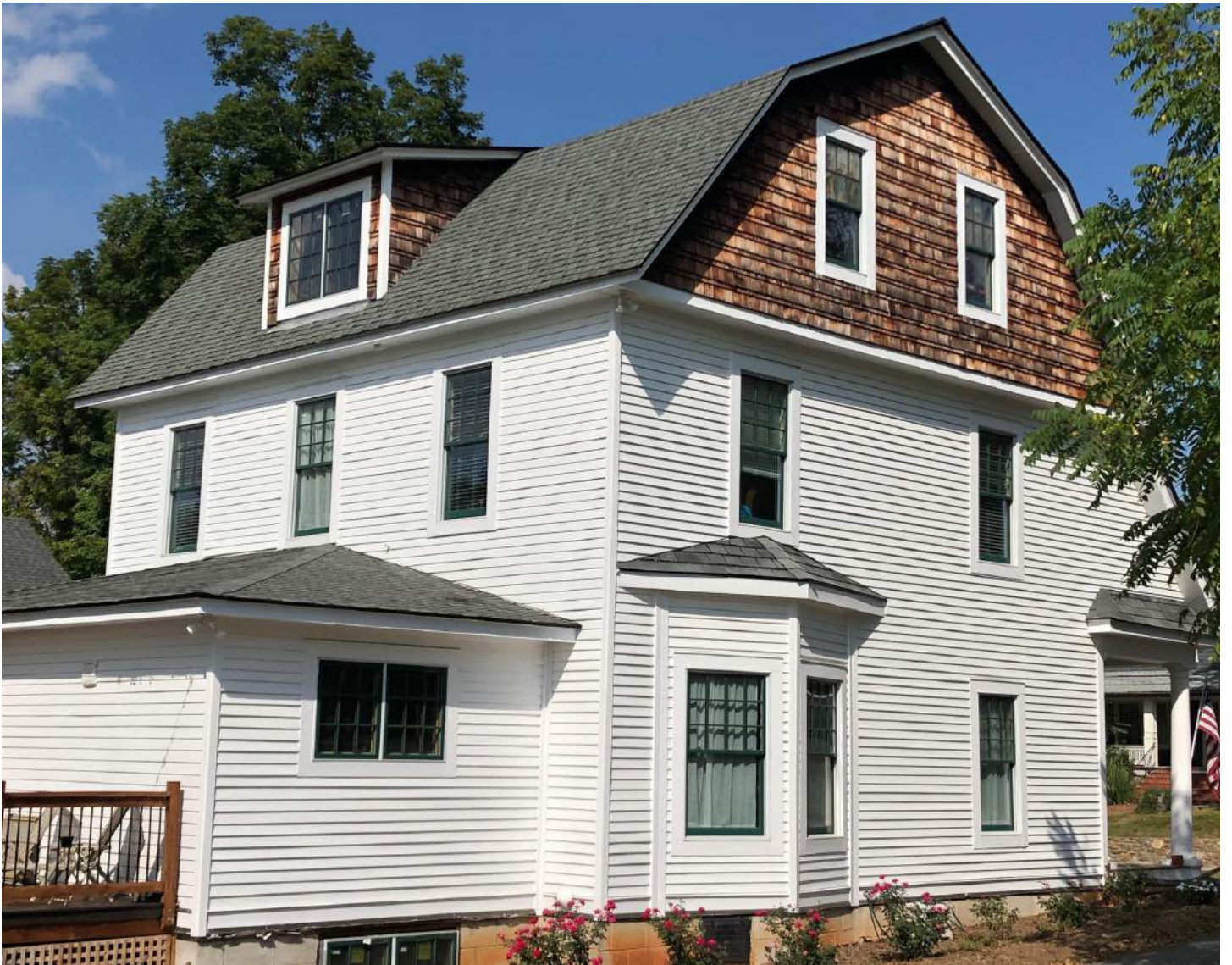
View from South Side
