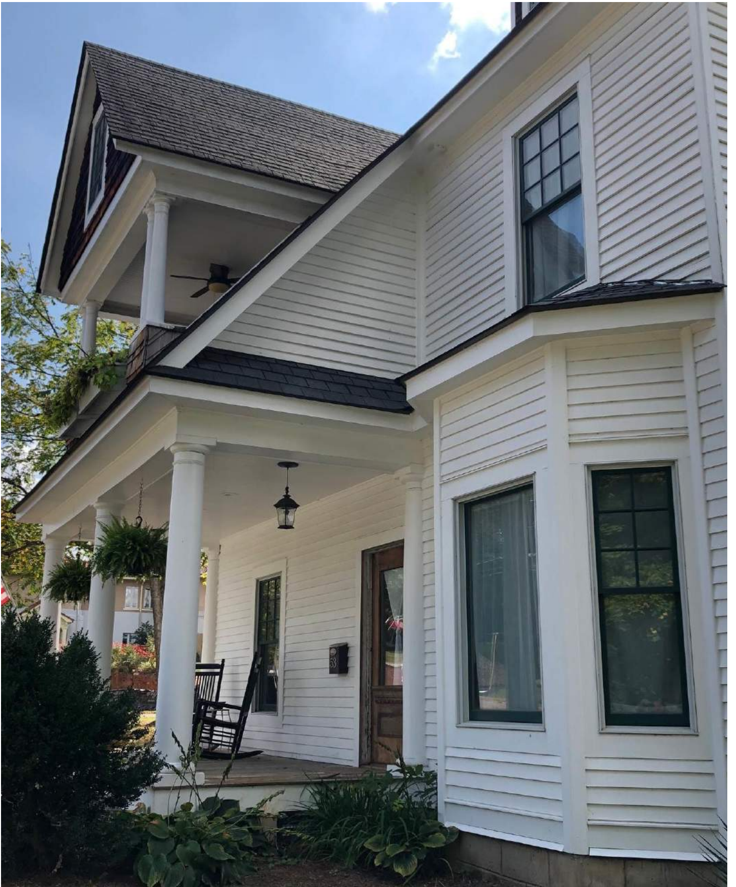
Closer View from Northeast Corner
