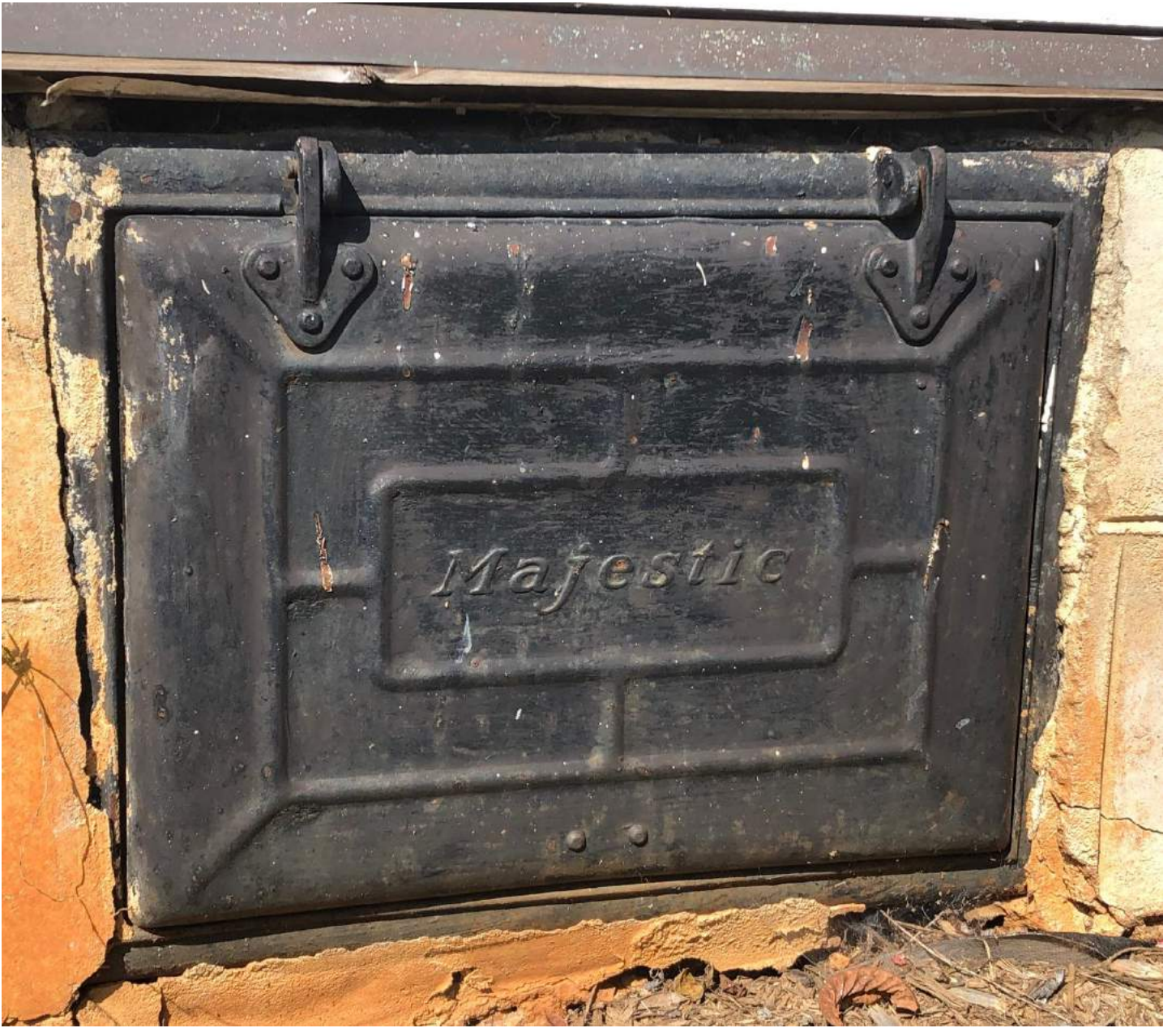
Coal Chute Door Beneath South Side Bay Window
