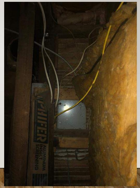
SERVICE ENTRANCE CABLE RUNNING THROUGH THE FLOOR JOIST TO A PANEL. THE FLOOR JOIST HAS FIRE DAMAGE.
