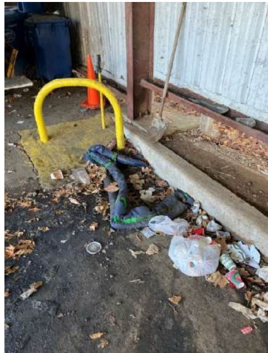
Public Works #4– Bay Inlet
