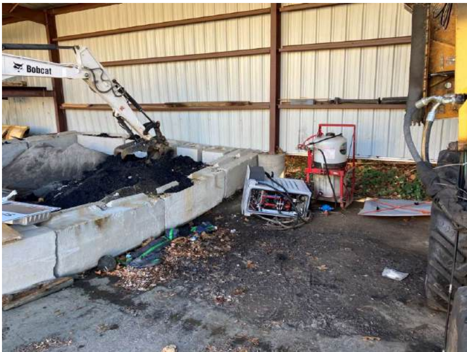
Public Works #6– Bay Inlet
