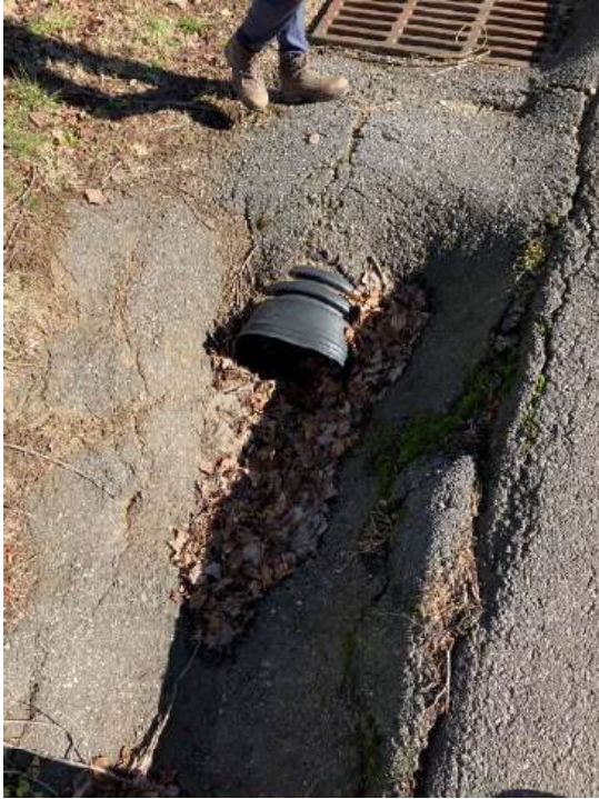
Hazelwood #1– Inlet and paved ditch on Westwood Circle
