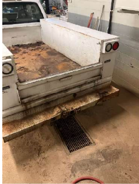
Public Works #2 – Floor Drain by eyewash station
