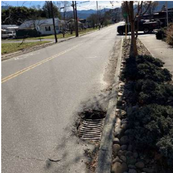
Fire Station #7– Brown Street inlet on west side
