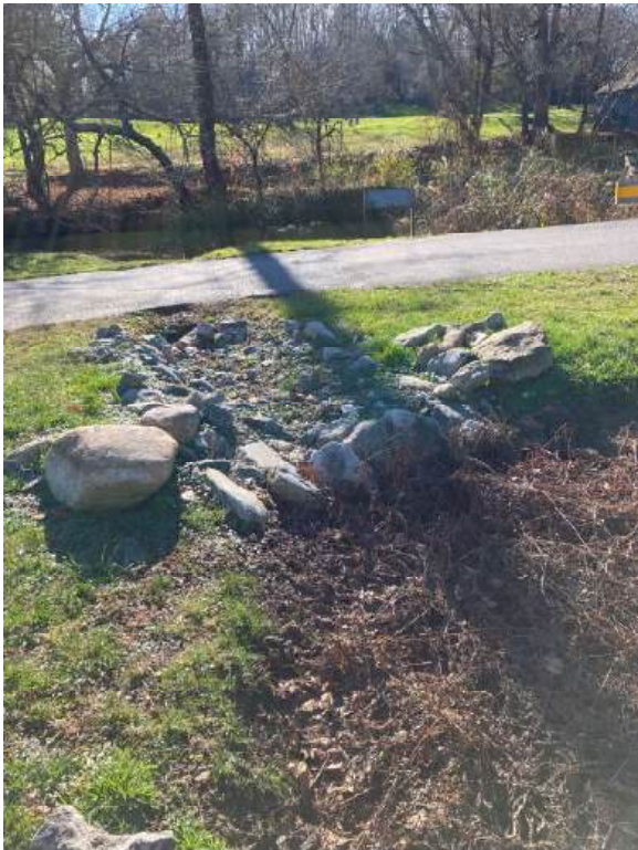
Greenway Rain Garden #2 – Outflow Channel
