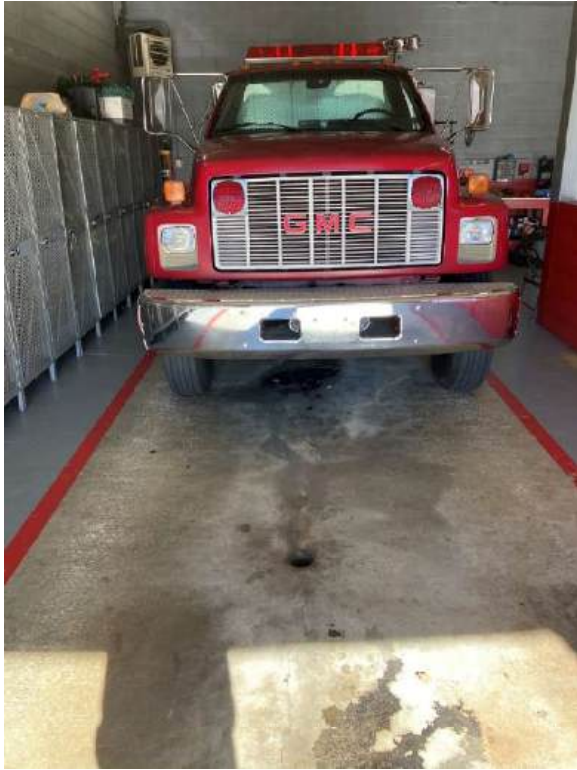
Fire Station #1– Parking Bay Inlet 1
