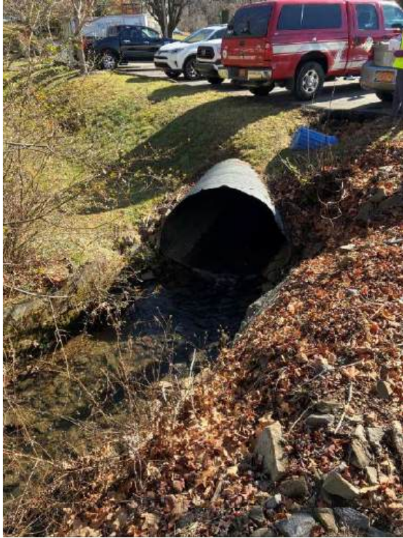
Fire Station #5– Pipe outlet on north side of parking lot
