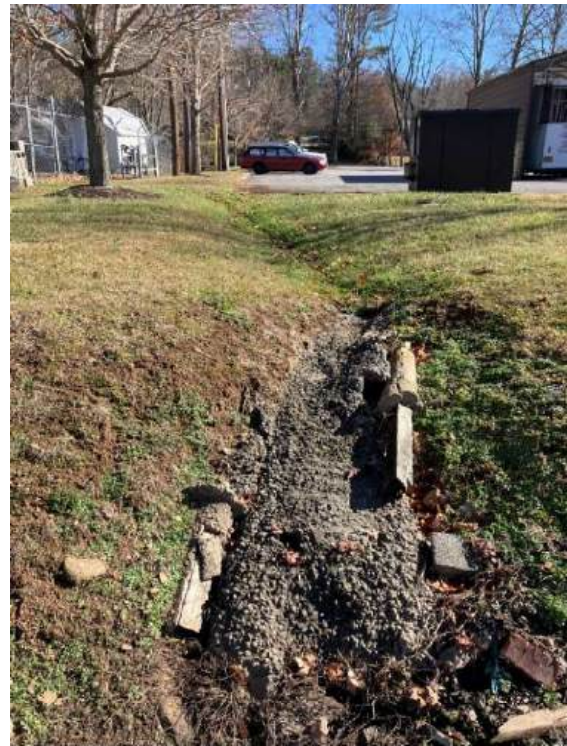
Fire Station #4– Outlet to Railroad Ditch
