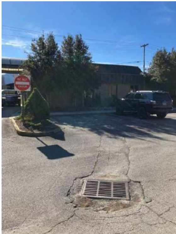
Fire Station #3– Parking Lot Inlet
