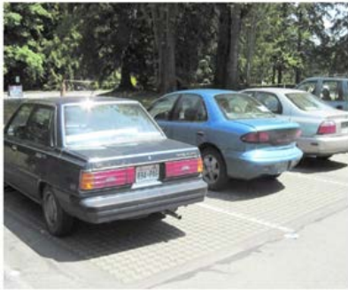
Pervious pavers and other pervious paving techniques allow stormwater to infiltrate into the ground below.
