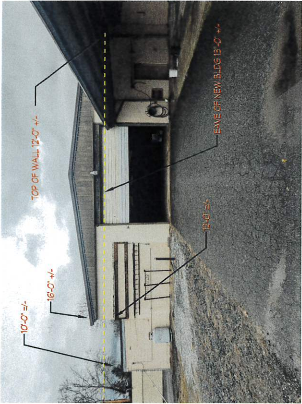
SOUTH ELEVATION BLDG B
