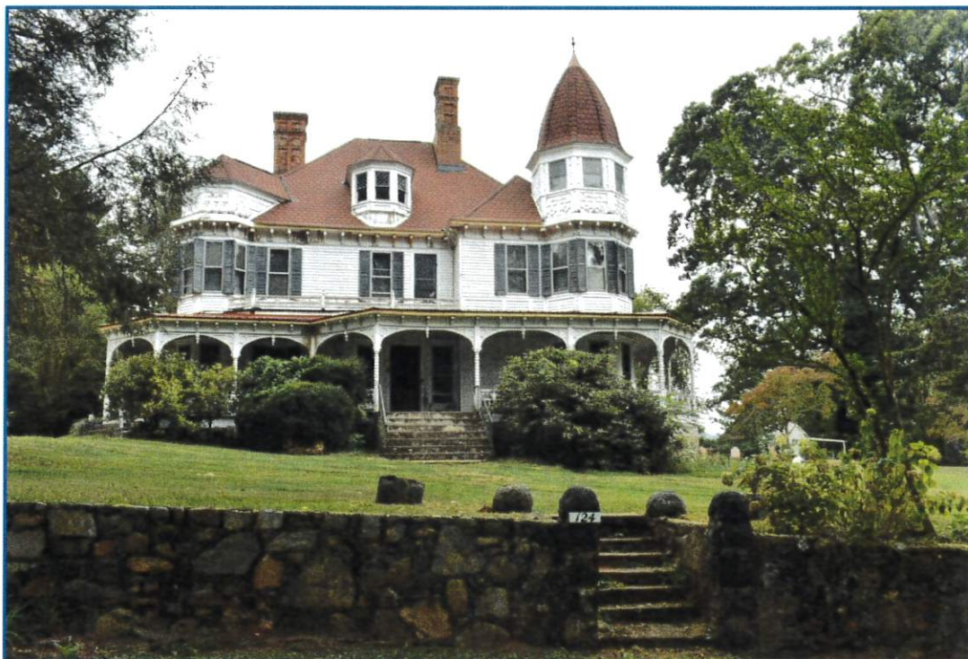
Photo 1. Façade, view to southwest
