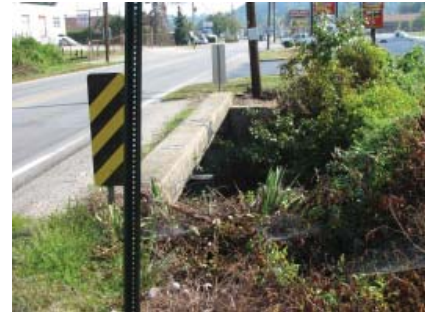
Allens Creek Bridge without railing and sidewalk.
