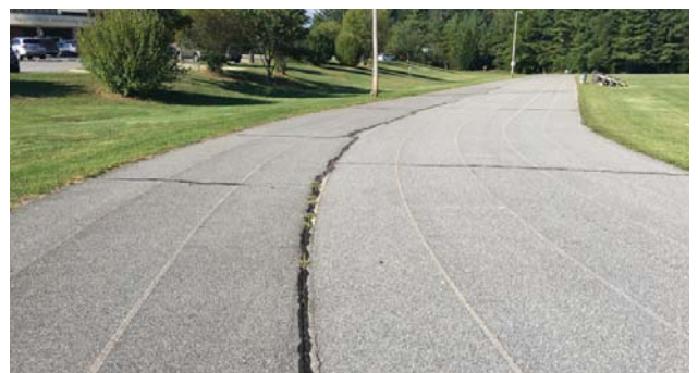
The existing walking track needs to be repaired
