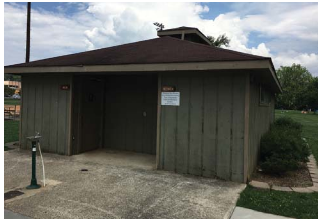
The existing restroom building should be renovated
