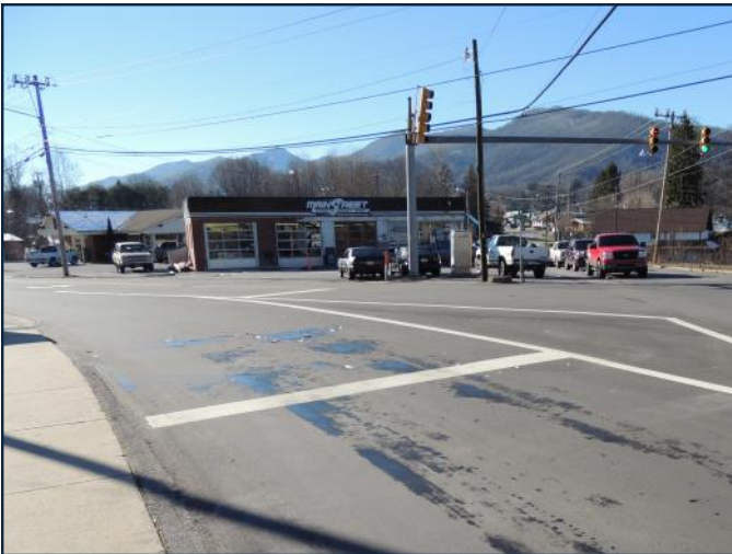
The Minor Realignment alternative would address the northbound right turn approach (shown in the foreground above) to create a 90-degree intersection. The major property impact would be to the auto repair shop (shown in the background above).
