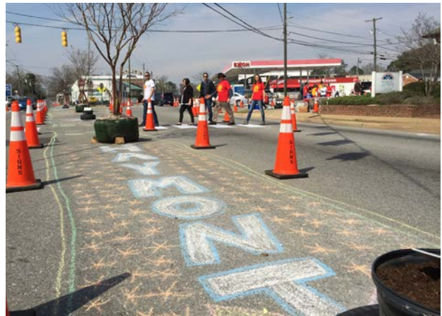
Temporary installation of a median and crosswalk is an example of tactical urbanism
