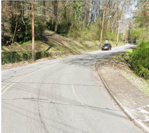
Figure 6 East Street Section 3 image looking from Happy Hollow Street
